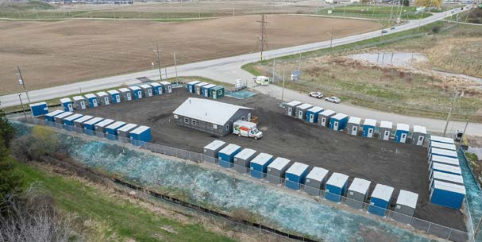
Figure 3: Outdoor Shelters at Erbs Road 33
